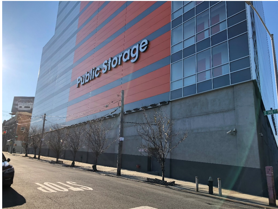
Photo 5: Southern adjoining property (looking southeast)
