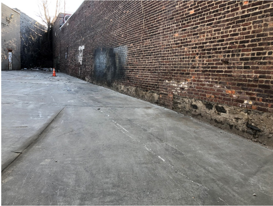
Photo 3: Northern Subject Property boundary and adjoining parking lot (looking east)
