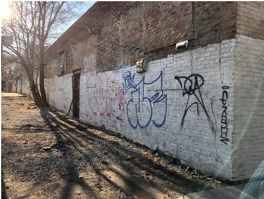
Photo 4: North adjoining warehouse (facing southeast)
