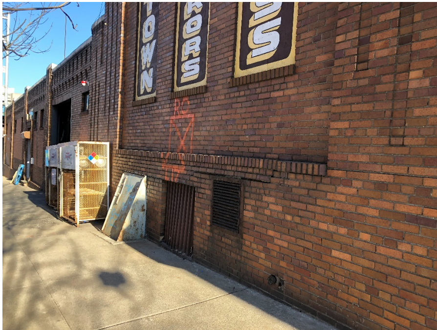
Photo 8: Fill port at eastern adjoining property (facing northwest)
